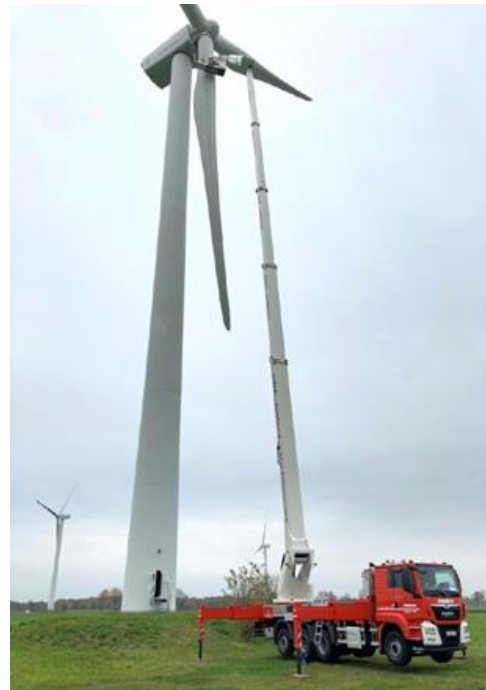
Fig. 2: Assembly of the tufts at great heights using a cherry picker
